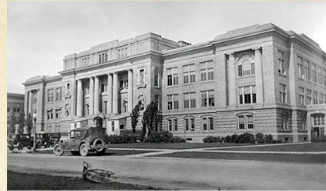
University Hall, originally constructed in 1915 is currently undergoing renovation.
